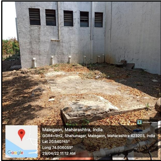
Soak pits for waste water collection from drainage
