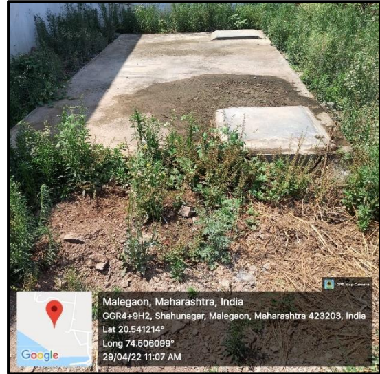
Soak pits for waste water collection from drainage
